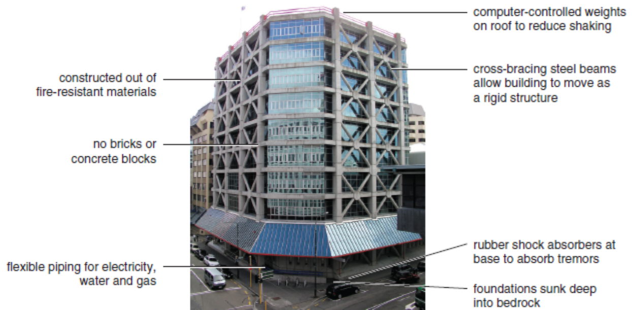
Figure 6.14 Some features of an earthquake-proof building.
