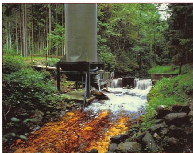
Figure 5.12 Controlled addition of lime to a stream in Sweden to neutralise the effects of acidity.
