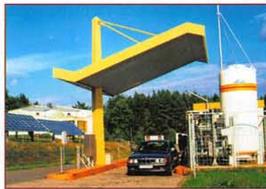
Figure 4.1 A car filling up with liquid hydrogen fuel at a solar hydrogen filling station. The hydrogen storage tank is on the right. Water is split into hydrogen and oxygen using power from the solar panels.
